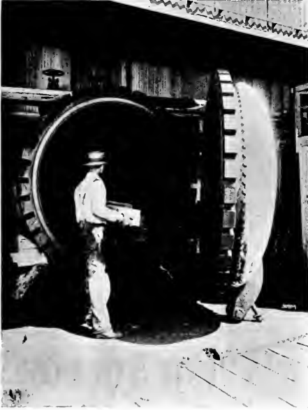
Testing Retort at Eagle Harbor
